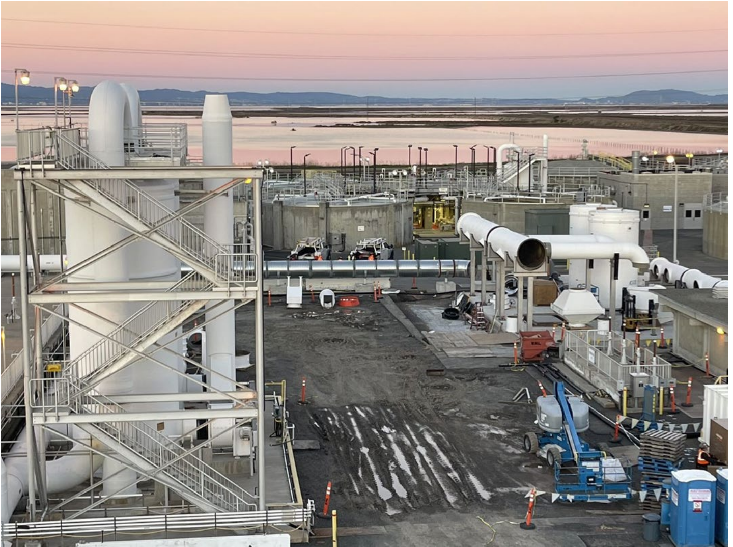
ETSU Aeration Basin Construction
