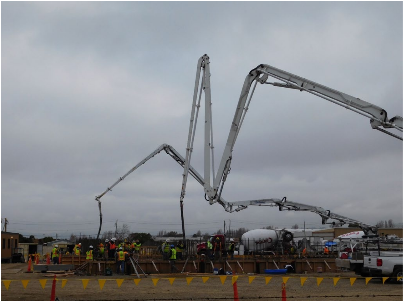
Pouring Concrete for the New Campus Building
