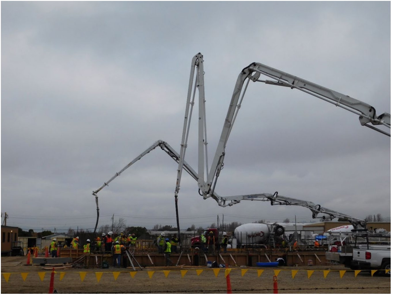
Pouring Concrete for the New Campus Building
