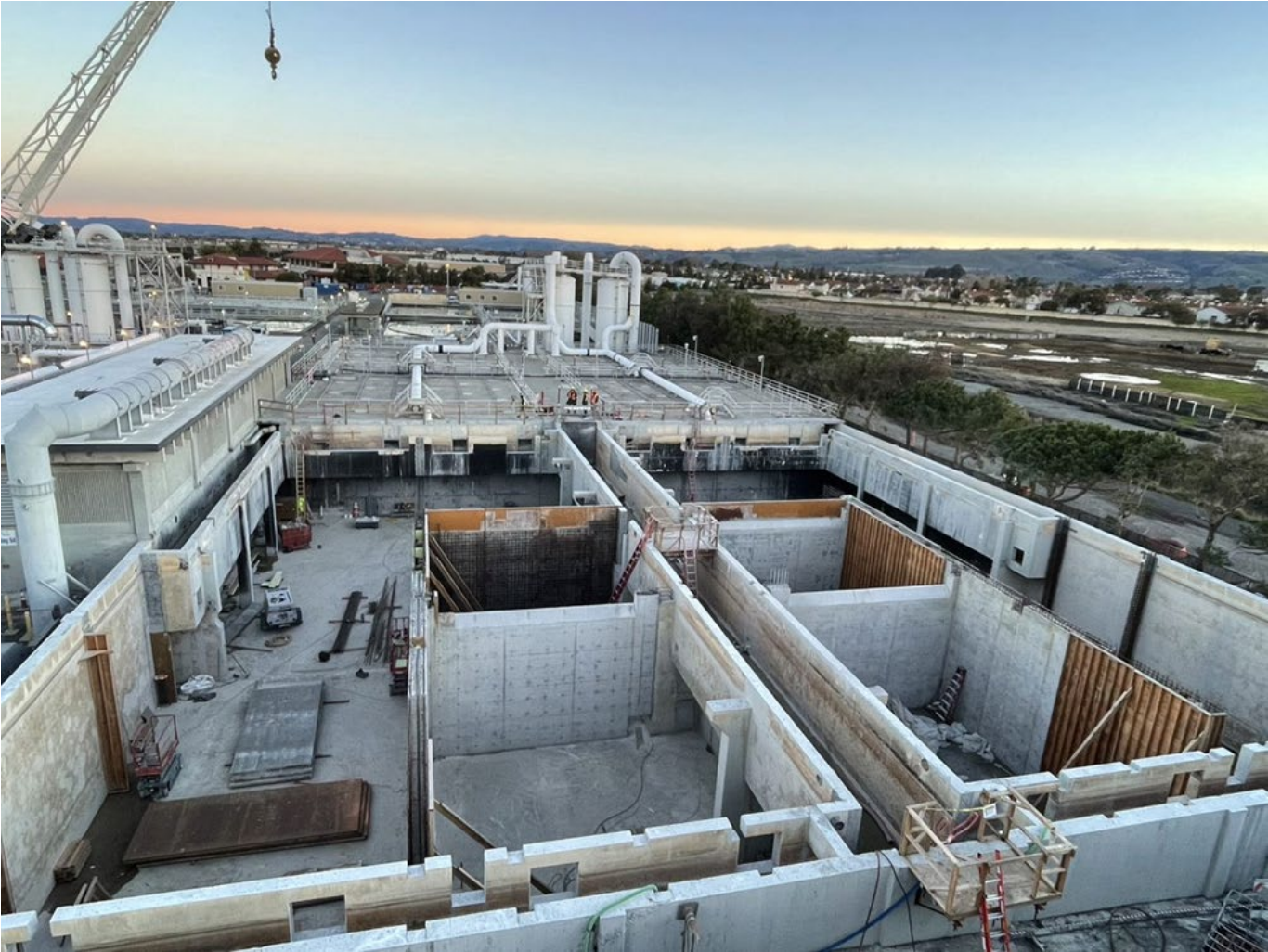
ETSU Aeration Basin Construction
