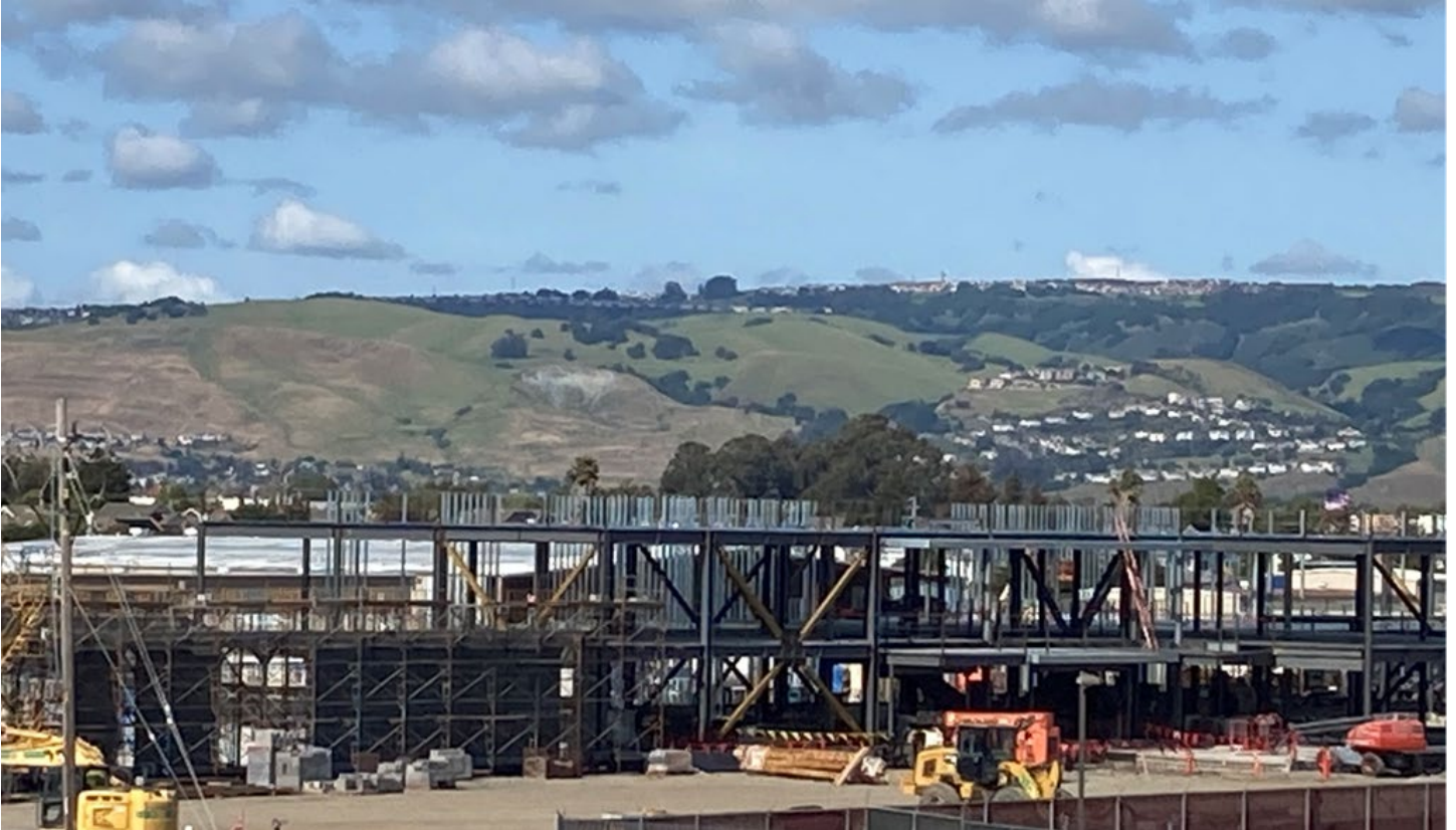
Structural Steel for the New Campus Building
