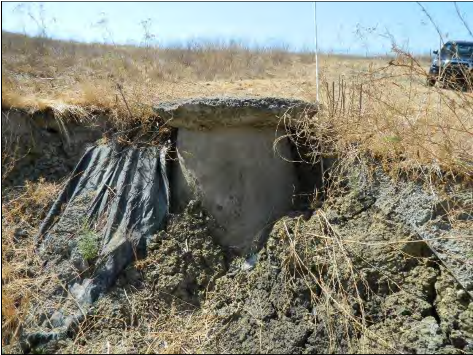
Figure 1 - Manhole G24006 - Looking South
