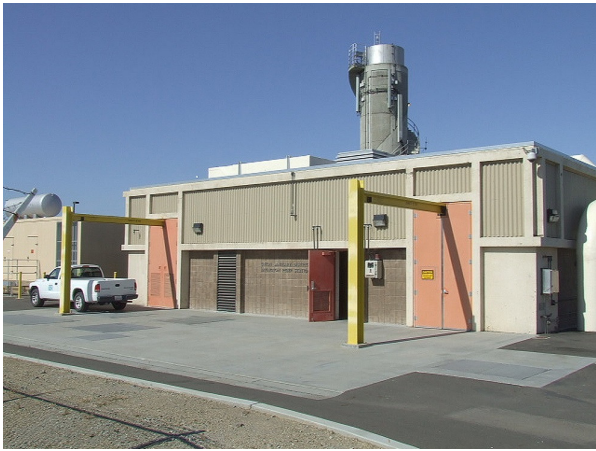
Irvington Pump Station
