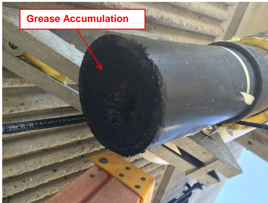
Photo 2 – PVC Pipe w/ Grease Accumulation
