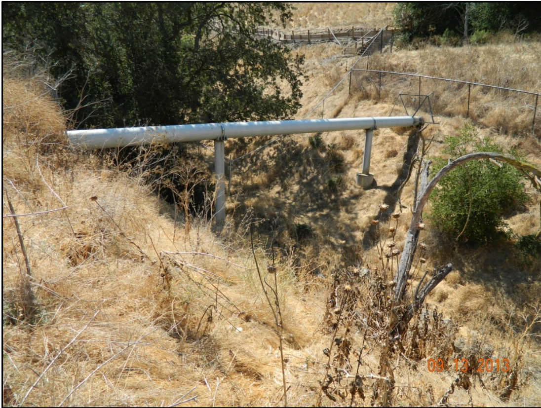
Photo 1 – Aerial Crossing (Pipe Bridge)
