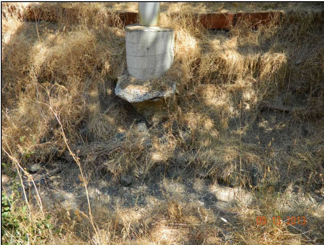
Photo 2 – Erosion At The Pipe Bridge's Eastern Foundation
