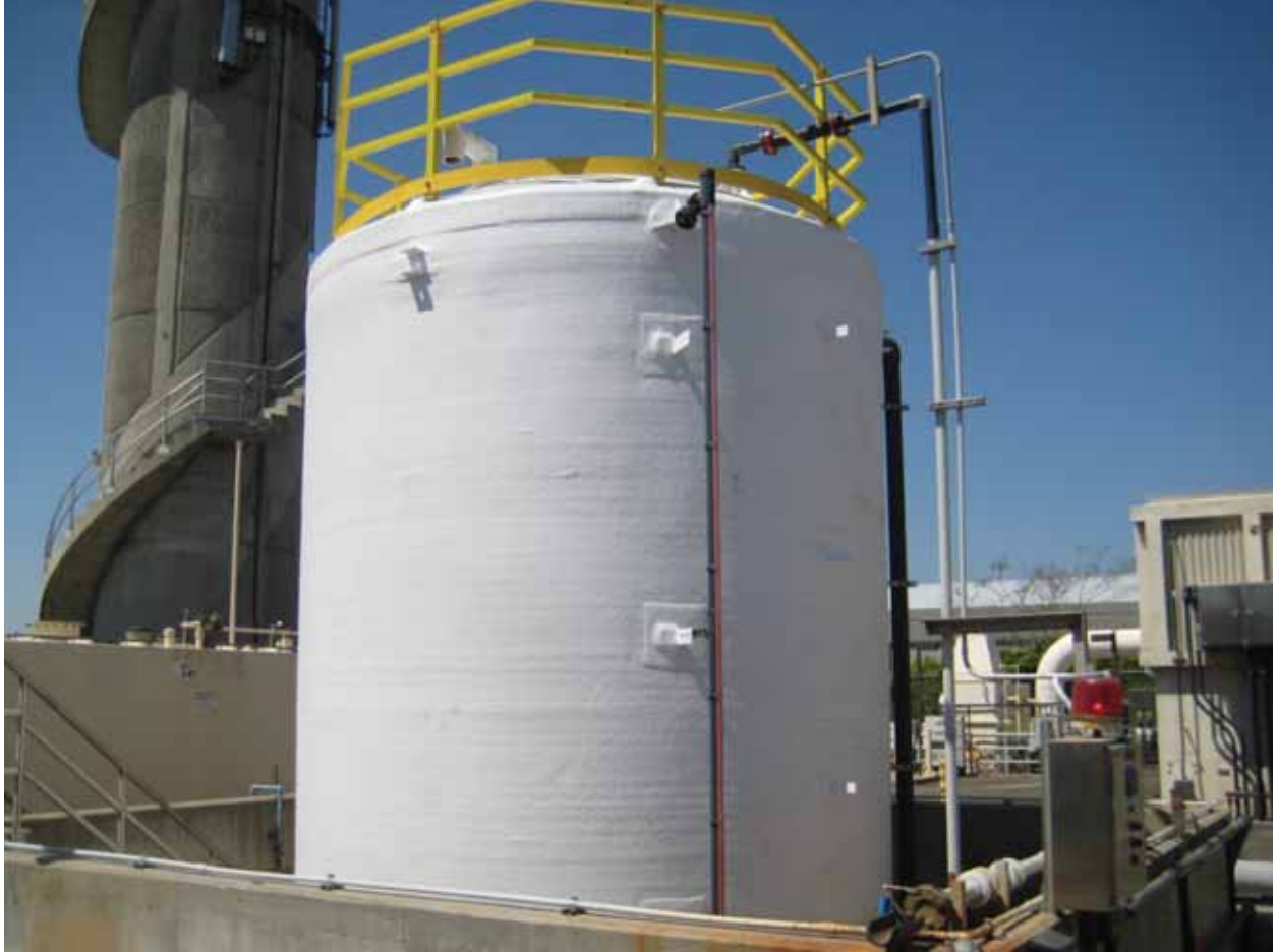
Ferrous Chloride Tank at Irvington Pump Station
