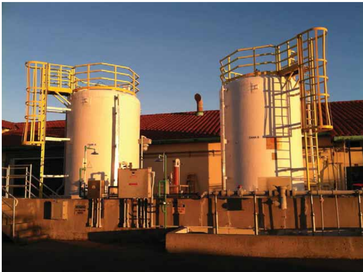
Sodium Hypochlorite Tanks A and B at Alvarado Wastewater Treatment Plant
