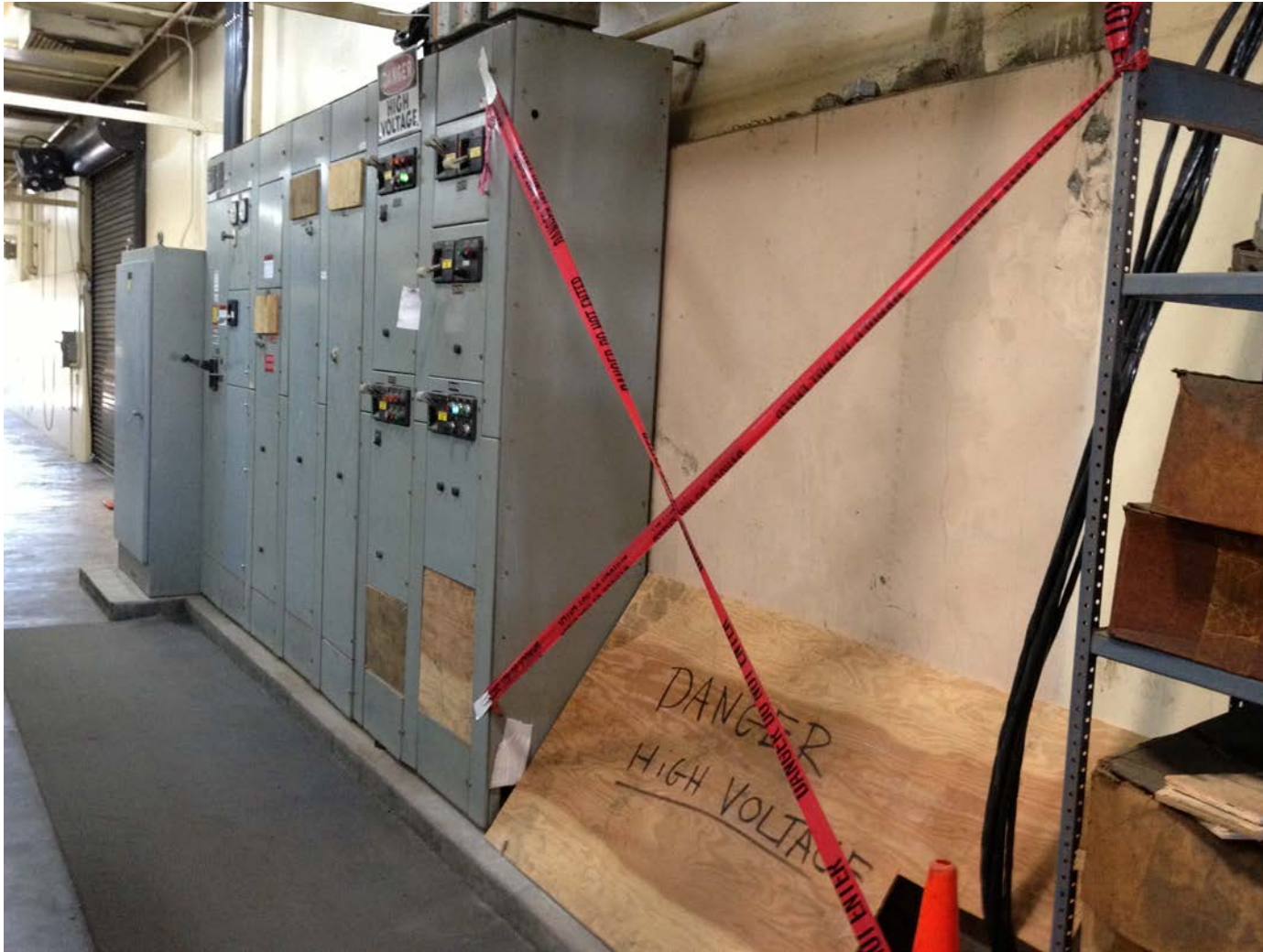
Old MCC 13 – East Aeration Blower Room. This photo illustrates the condition of the Westinghouse MCCs installed in the mid 1980's.
