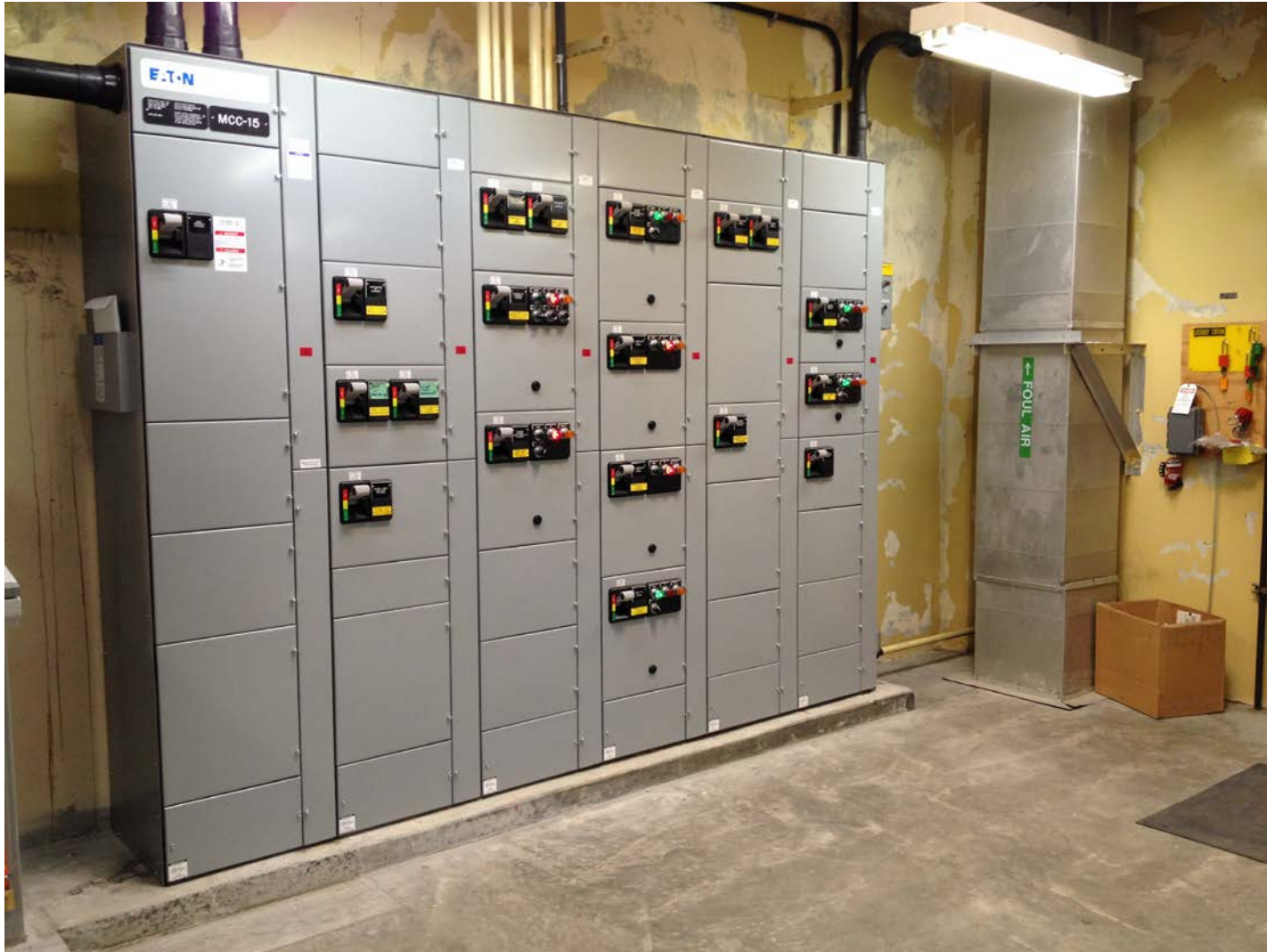
New Motor Control Center No. 15 – Alvarado Pump Station
