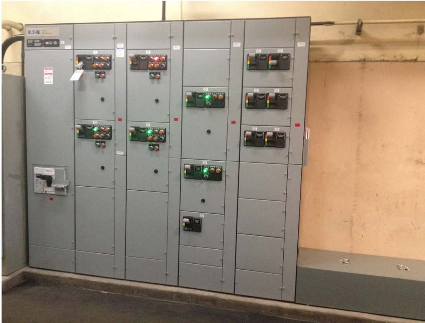
New Motor Control Center No. 13 – East Aeration Blower Room
