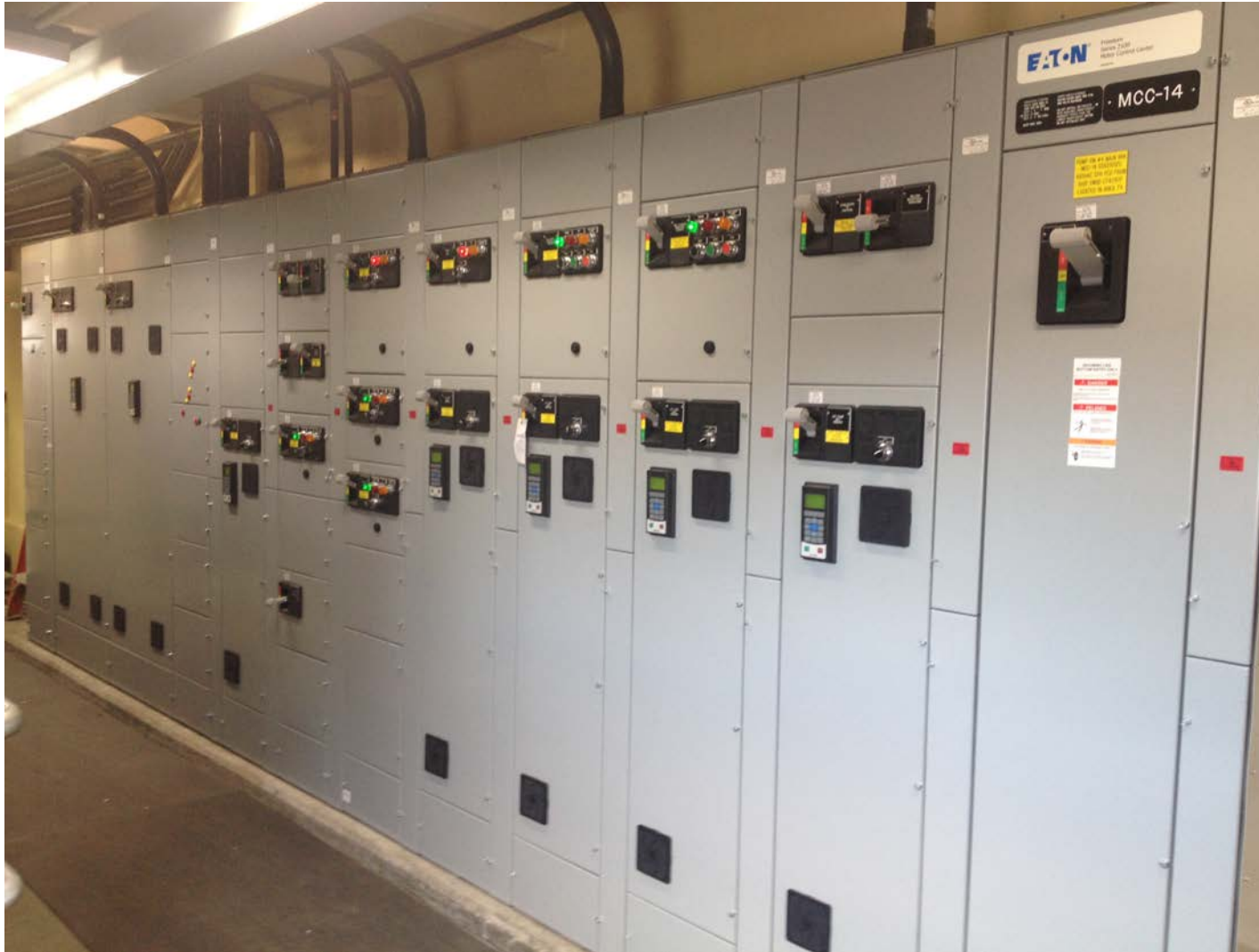
New Motor Control Center No. 14 – Sludge Pump Room No. 4 (across from MCC No. 27)
