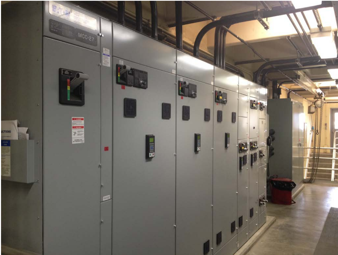
New Motor Control Center No. 27 – Sludge Pump Room 4 (across from MCC No. 14)
