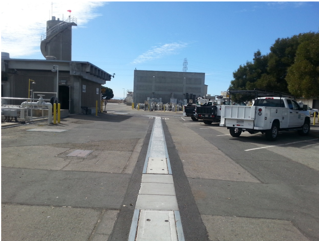
Figure 9 – New Precast Concrete Trench Between the MSB and the Water Champ Chemical Mixer Area
