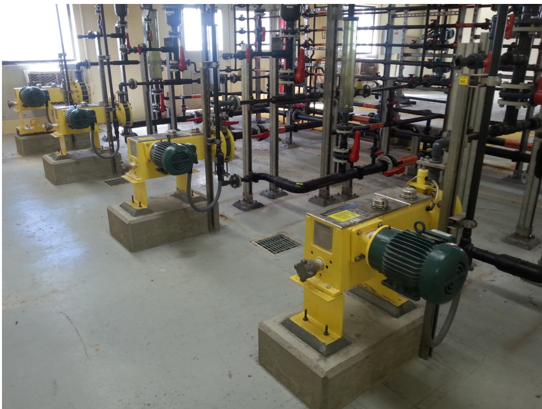
Figure 5 – New OCB Chemical Metering Pumps, piping and pipe rack
