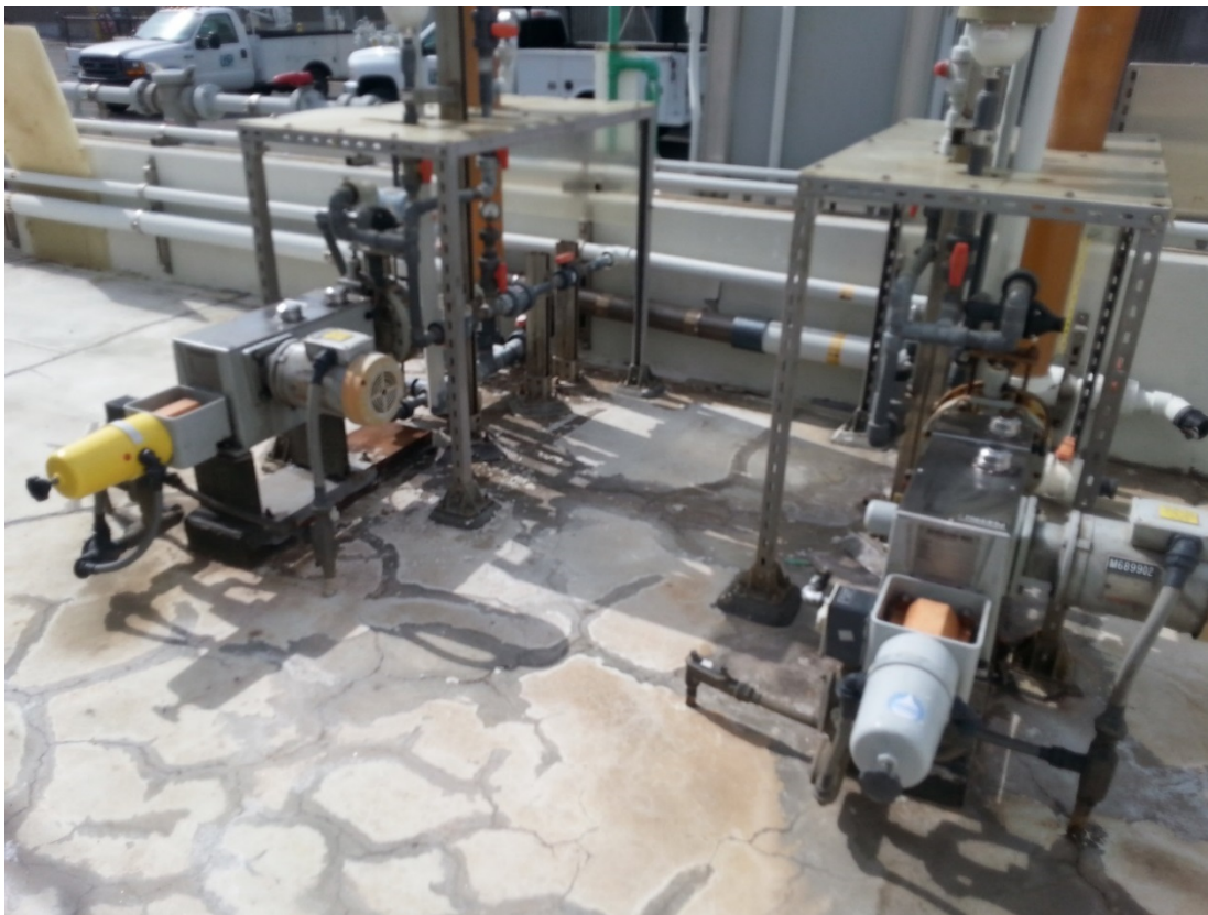
Figure 6 - MSB Chemical Metering Pumps and Piping before the Project
