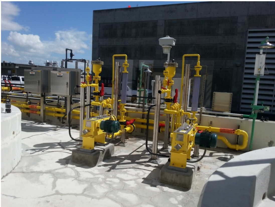
Figure 7 – New MSB Chemical Metering Pumps and Piping
