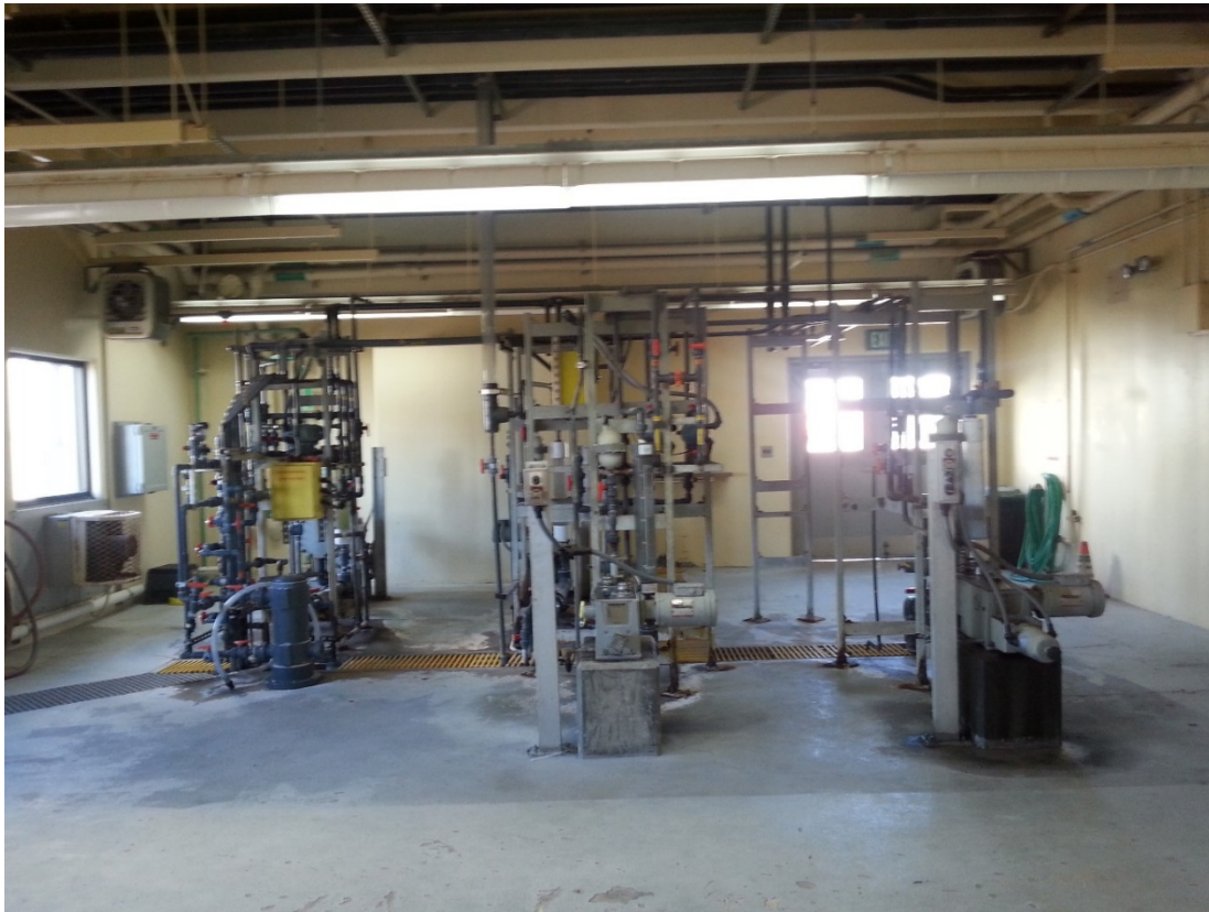
Figure 4 - OCB Chemical Metering Pumps and piping before the Project
