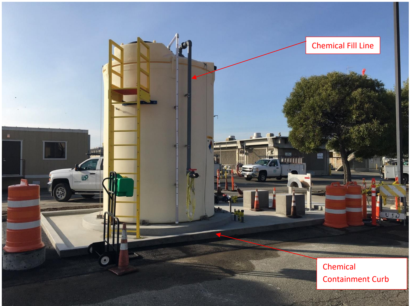
Figure 3 – New Calcium Thiosulfate Chemical Tank and Concrete Pad
