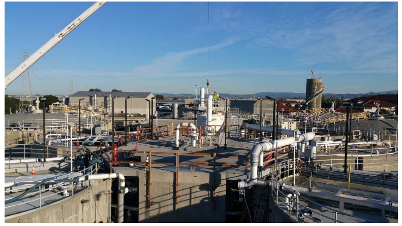
Digester maintenance and rehabilitation
