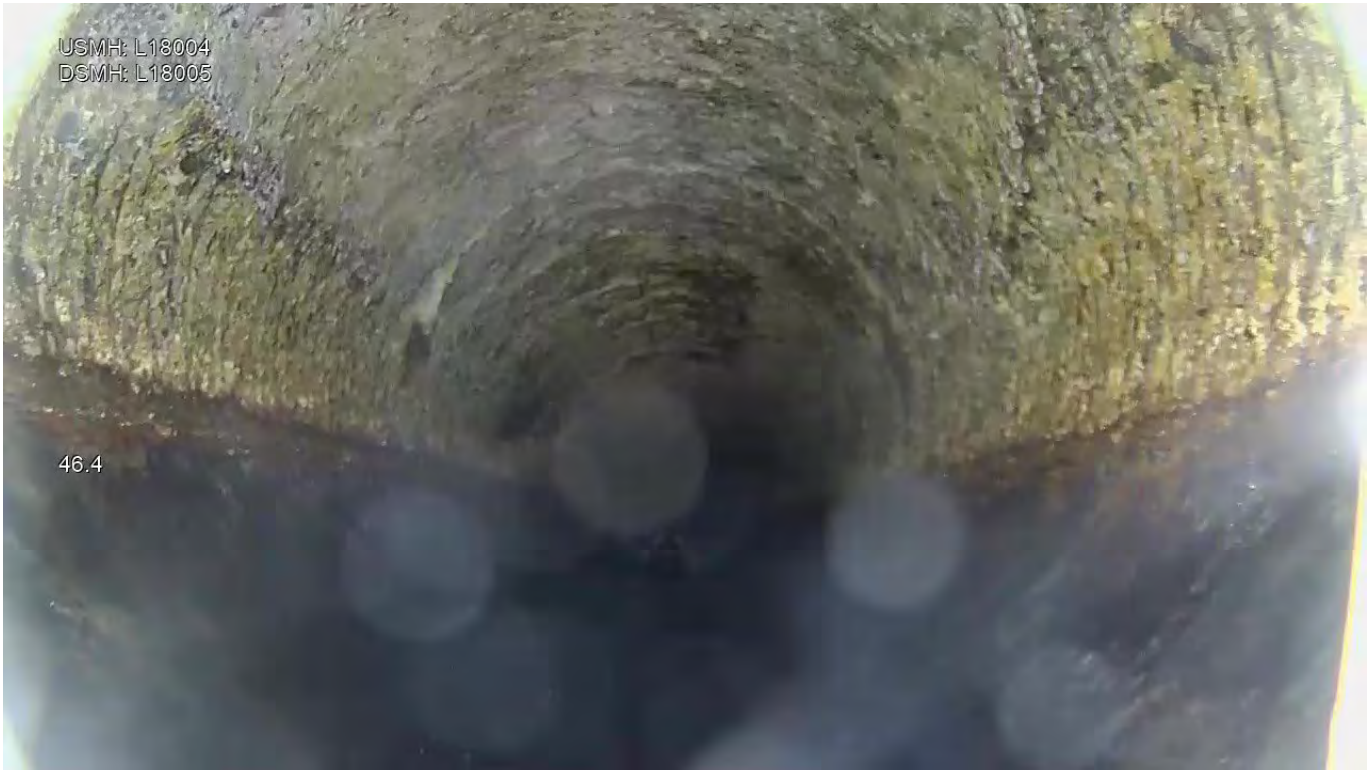
Figure 8 – Before photo of Reinforced Concrete Pipe
