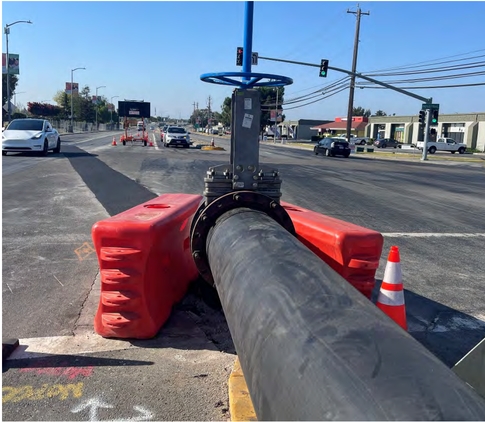
Figure 4 – Bypass Piping Transitioning from Median to Below Grade
