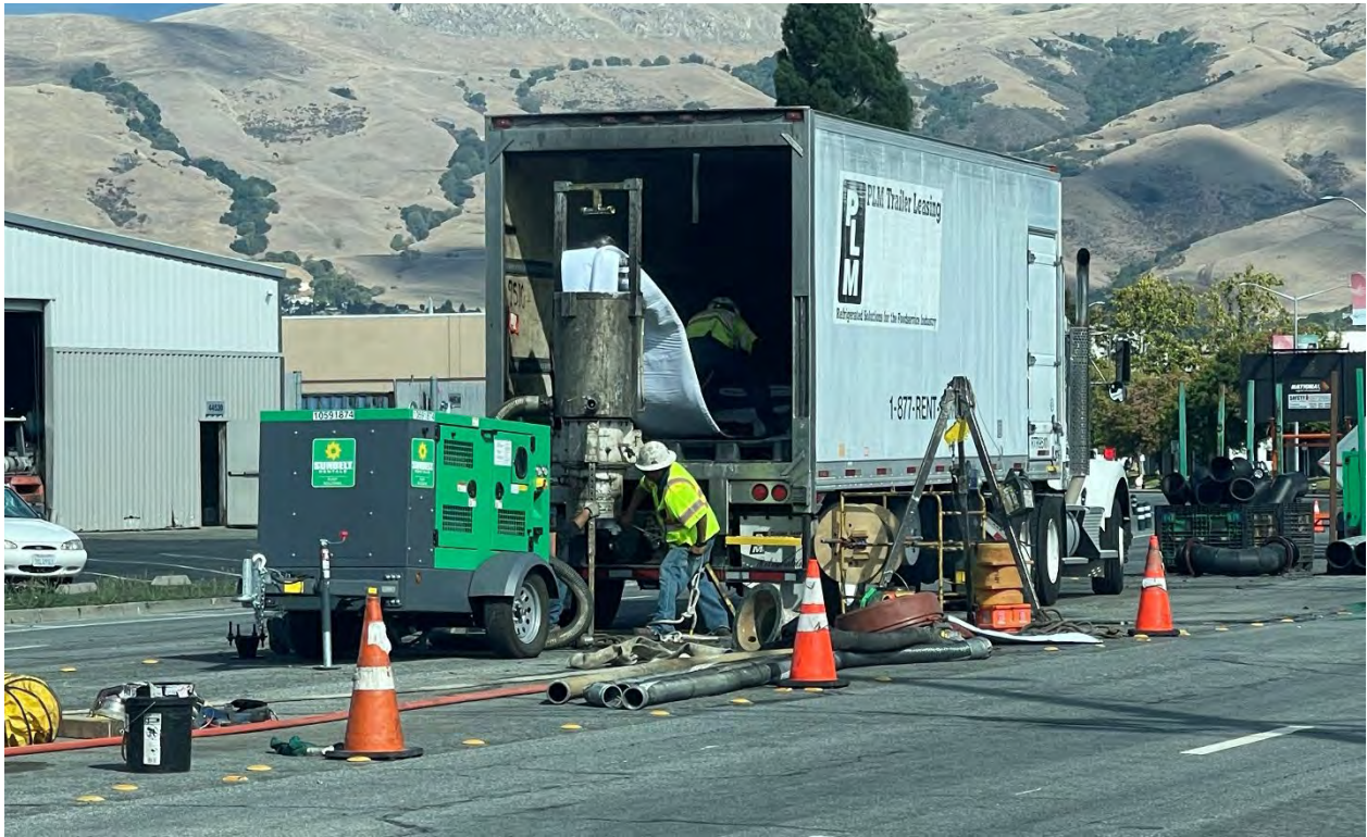
Figure 6 – Installation of Cured-in-Place Pipe Liner
