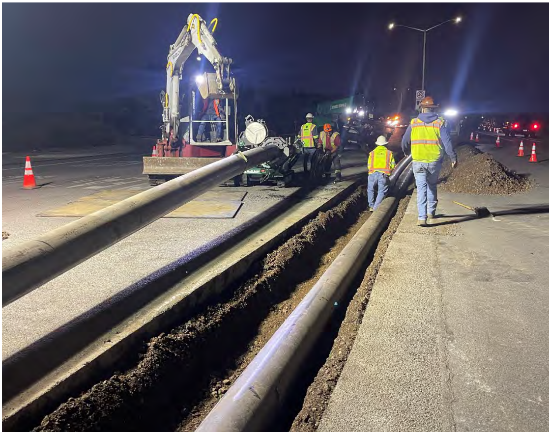
Figure 3 – Installation of Bypass Piping at Intersection
