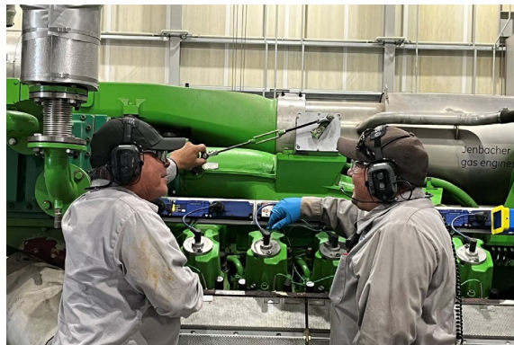
Mechanics working on the cogeneration engine
