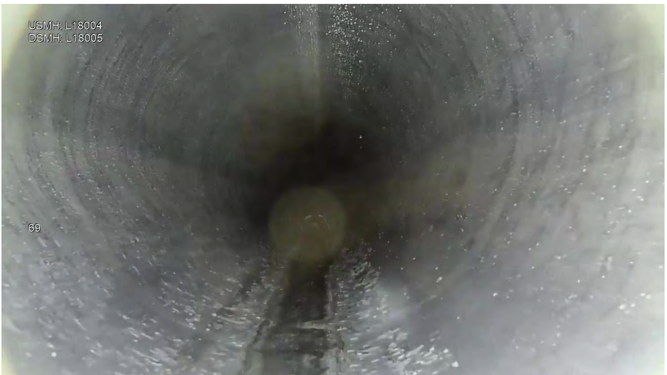
Figure 9 – After photo of Cured-in-Place Lined Pipe
