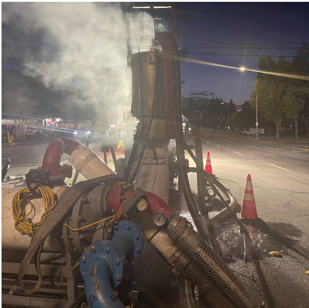
Figure 7 – Heating of Cured-in-Place Pipe Liner
