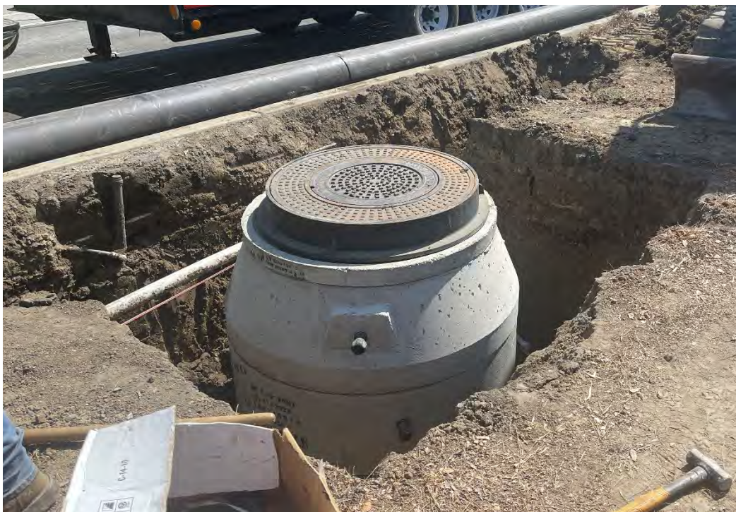
Figure 11 – After Photo of New Manhole
