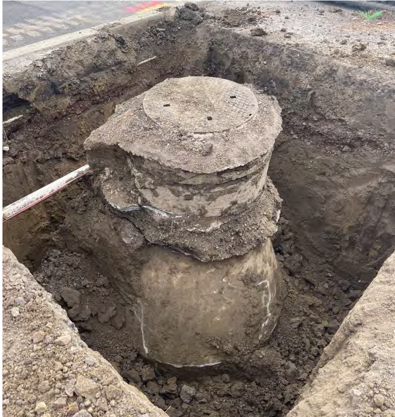
Figure 10 – Before Photo of Existing Manhole
