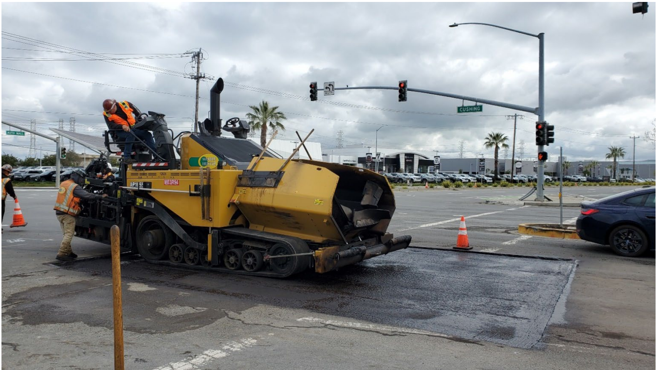
Figure 4 – Final Pavement of Entire Area
