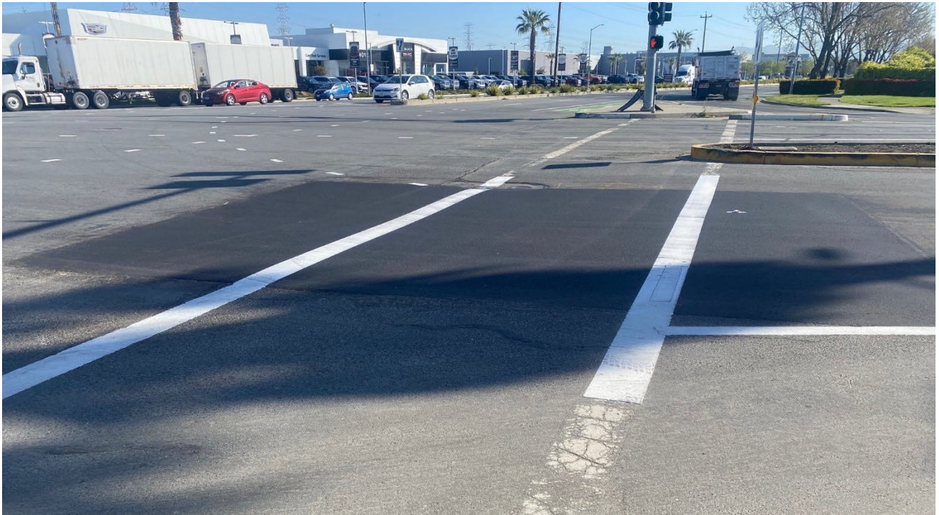
Figure 5 – Completed Repair of Intersection
