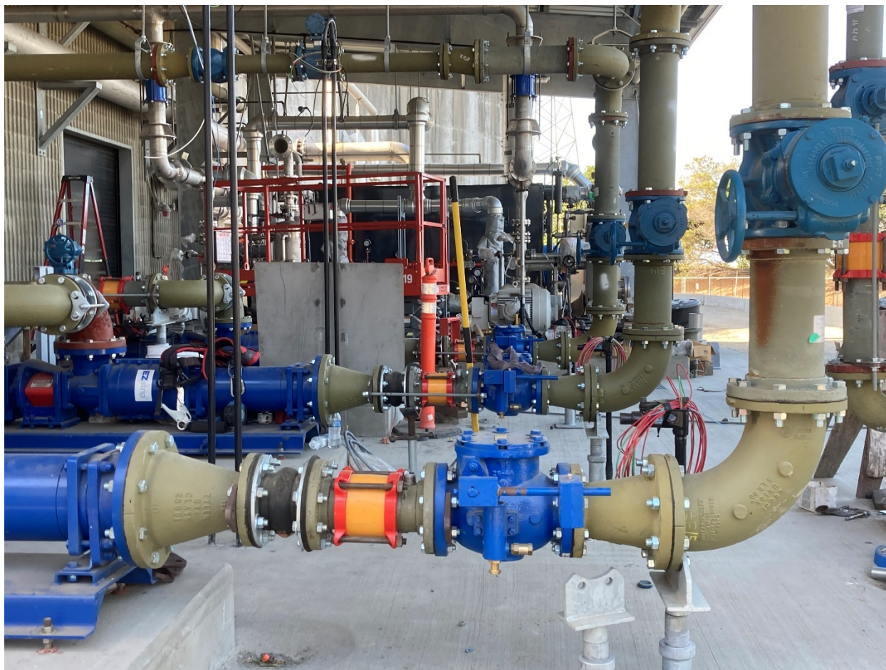
New Control Pumps and Piping for Digester 7
