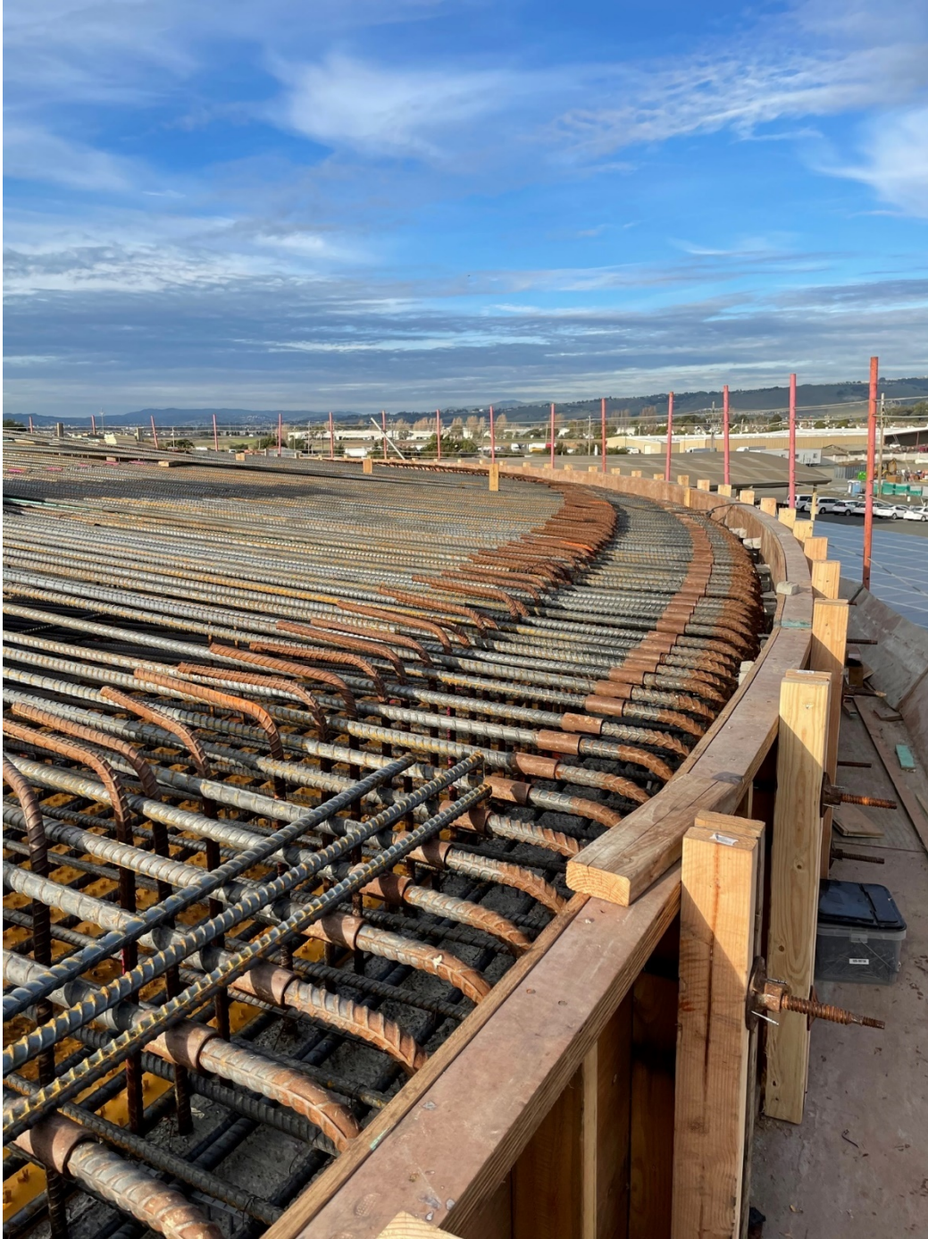
Rebar Layout Digester 7 Roof
