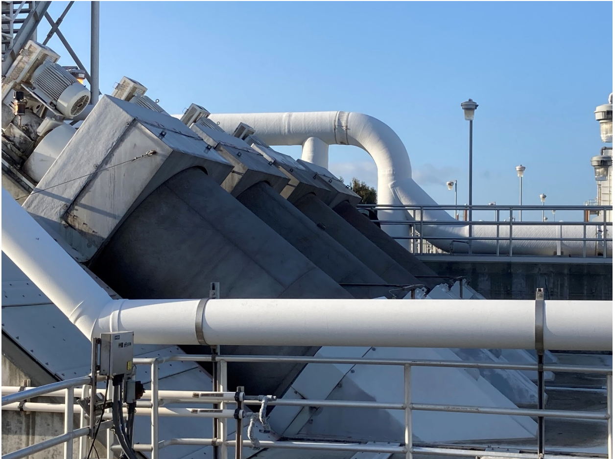
Primary Effluent Pumps for the Aeration Basin
