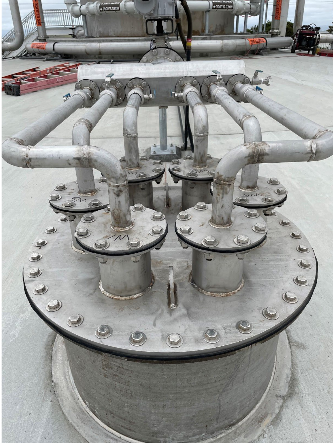
Gas Lance Mixing Header – Digester 7
