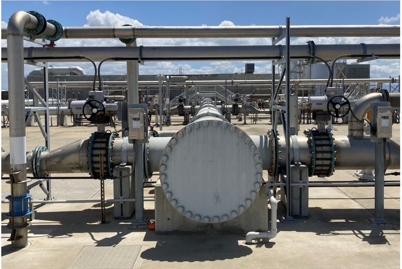
Air Piping System for Aeration Basins 5 Through 7
